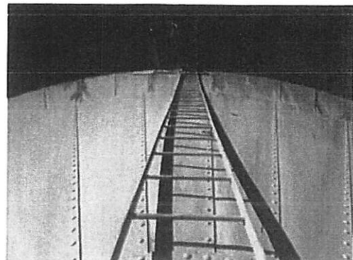
Roof exterior: showing revolving ladder to be intact and in good structural condition.
