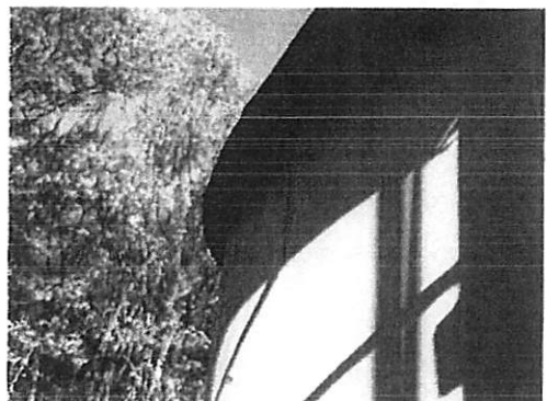
Shell exterior: showing rust staining weeping down from the unsealed roof to shell junction.
